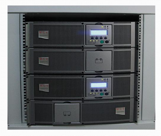
**UPS MGE Pulsar** MX 5000 RT3U **Output Power:** 5000 VA(4500W), Supported Output Voltage up to 240V(1) - 280V(3)with 50/60Hz; Backup/Time 62 min
