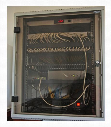
Communication rack is installed at each floor supplied with UPS: **Output Power 600** VA(360W); Supported output voltage up to 230V(1) with 50/60Hz and Cisco Switch 500 10/100 Mb/s providing intranet.
